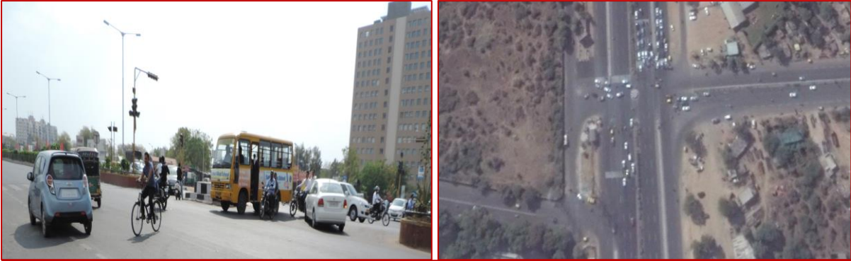
Misaligned four way intersection with no proper signage and inoperative traffic signal
