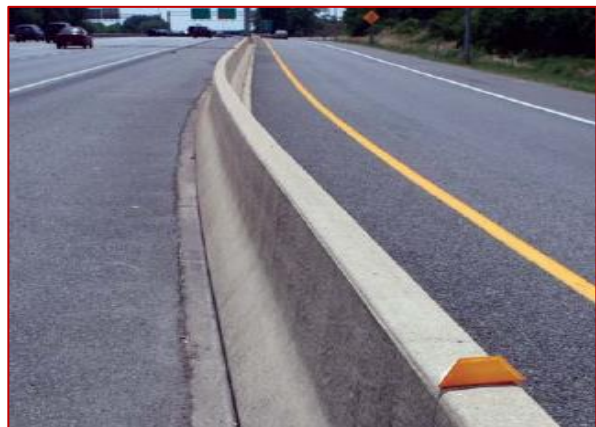
Concrete Jersey barrier
